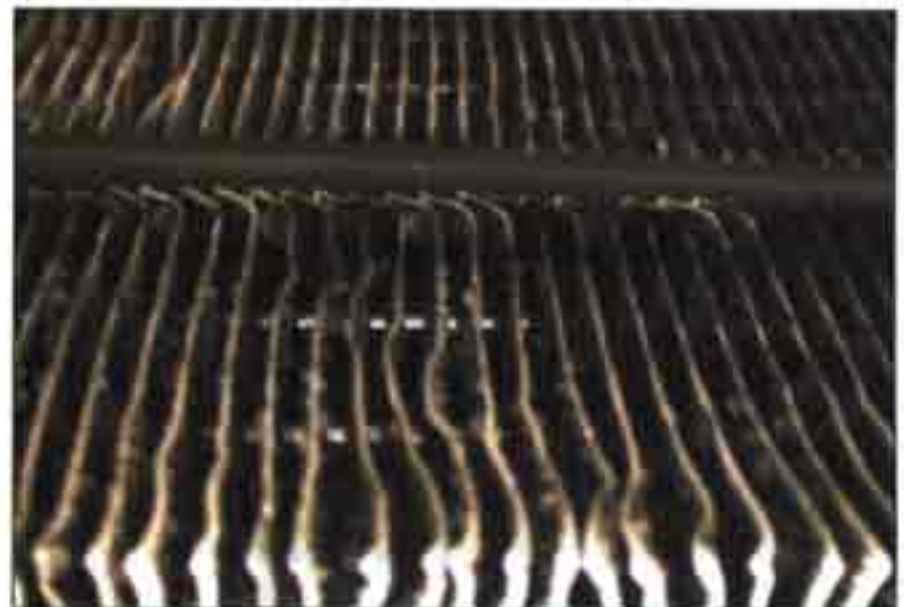
A reach-in freezer evaporator coil is shown after 16 hours of operation at -14.5° F. The absence of frost bridging between fins extends periods between defrost cycles.
